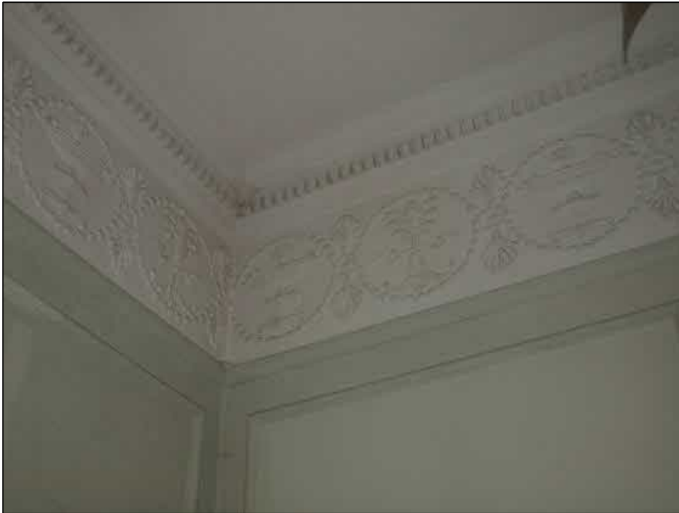
Plate 64: Room 17 plaster frieze
