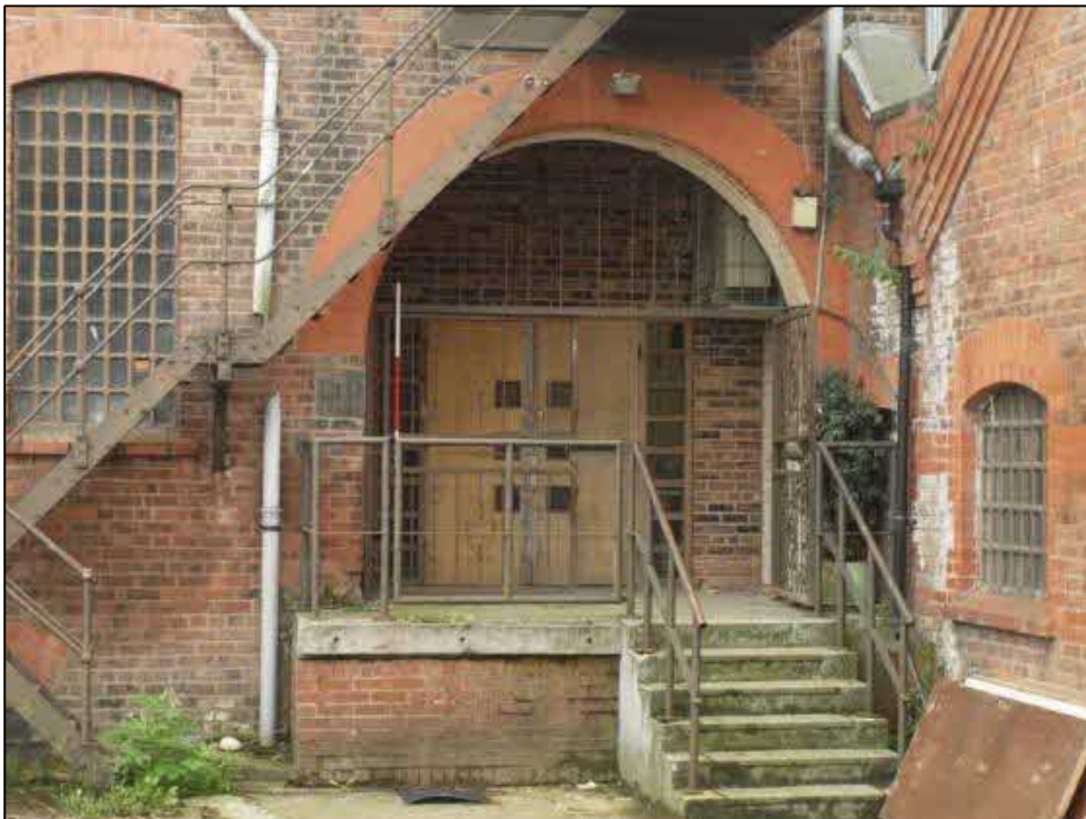
Plate 12: Loading entrance with inserted platform and doorway
