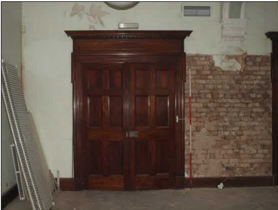
Plate 55: Detail of doorway to room 14
