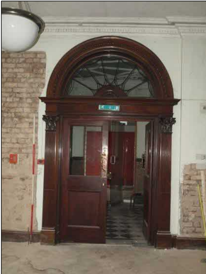
Plate 56: Detail of doorway to entrance lobby (room 9)
