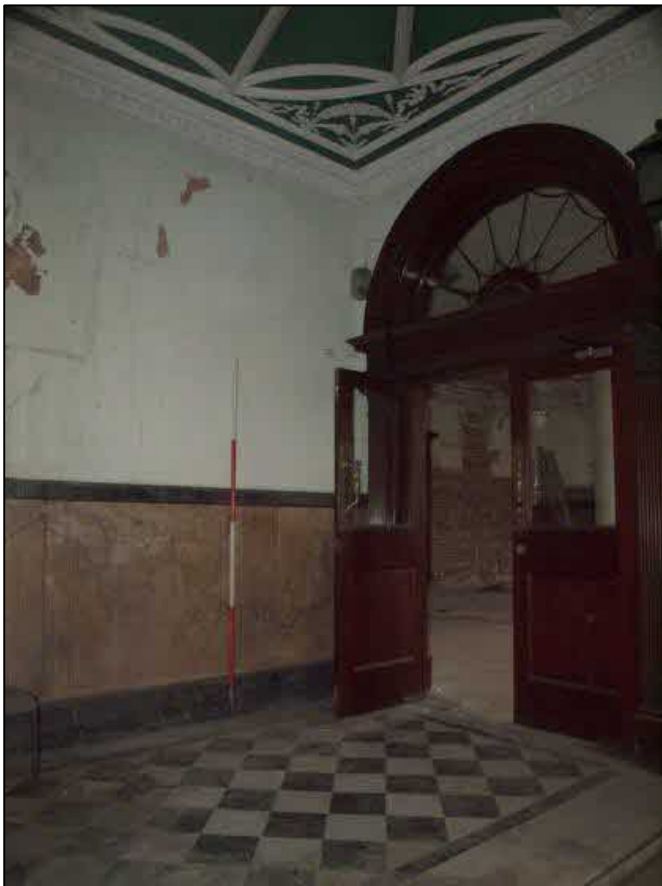
Plate 37: Room 9, main entrance lobby showing doorway to room 15
