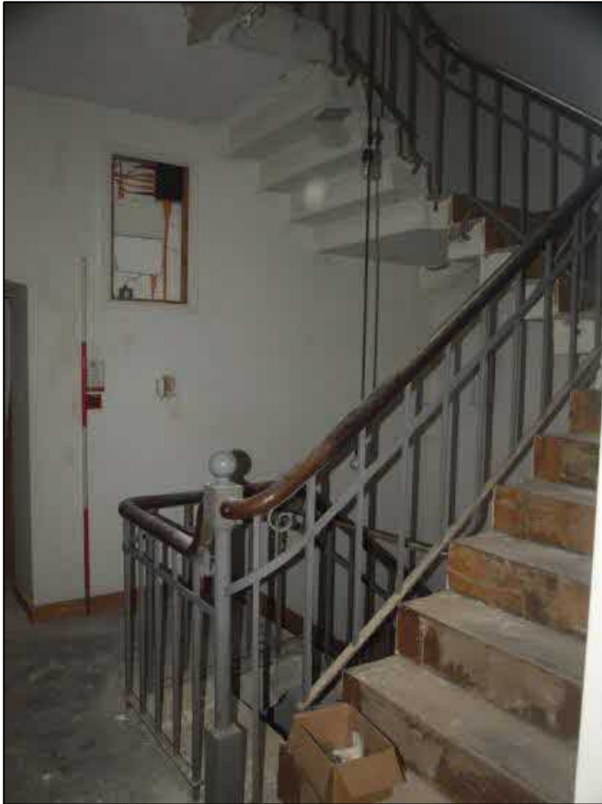
Plate 97: Main staircase room 1
