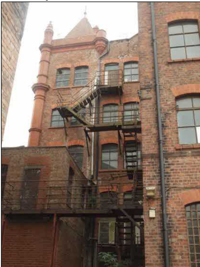
Plate 16: Bays 10 and 11 upper floors
