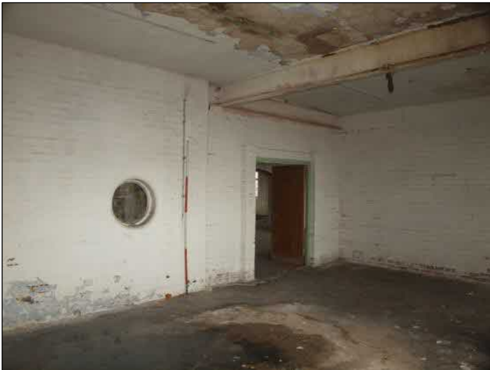
Plate 117: Room 3 showing blocked circular window
