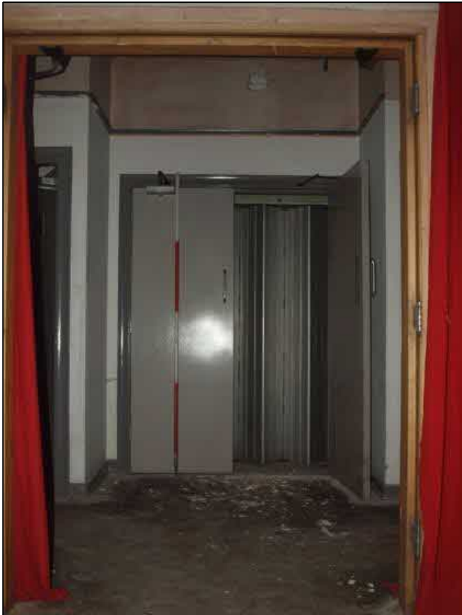
Plate 46: Room 12 showing inserted lift
