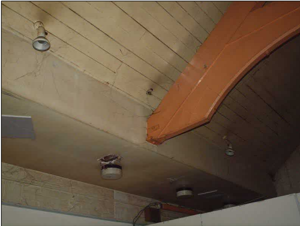
Plate 164: Truss running into boxed in area
