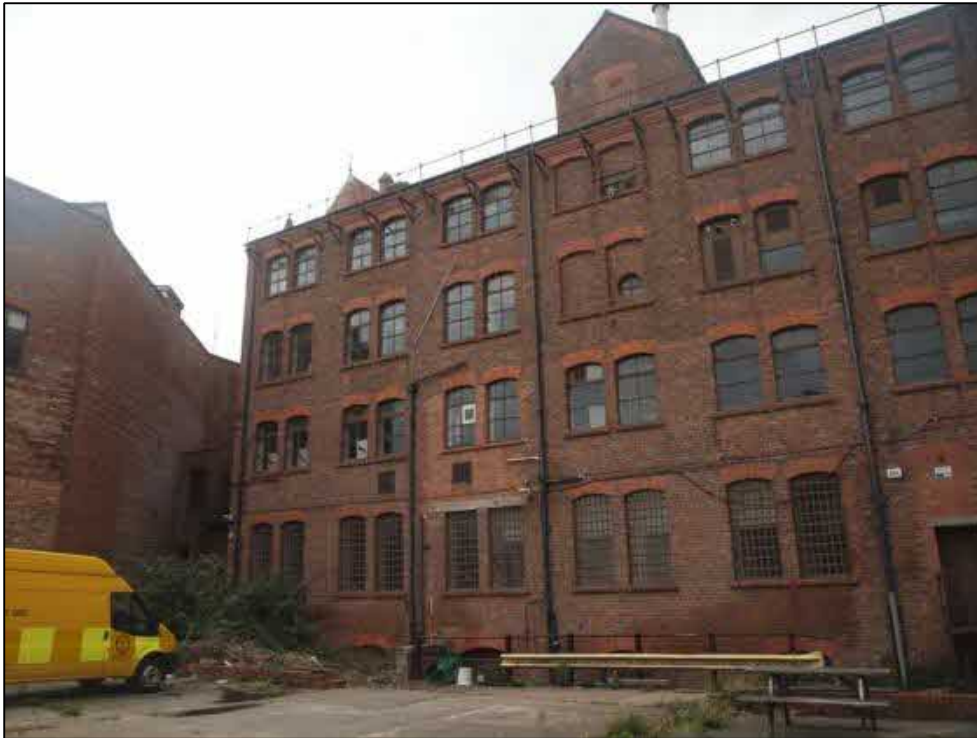
Plate 11: General shot of rear elevation
