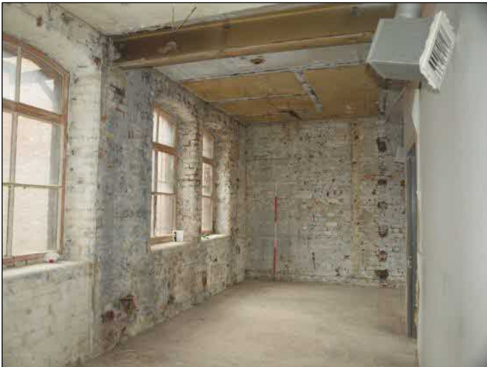
Plate 100: Room 2 showing ceiling scars of removed walls
