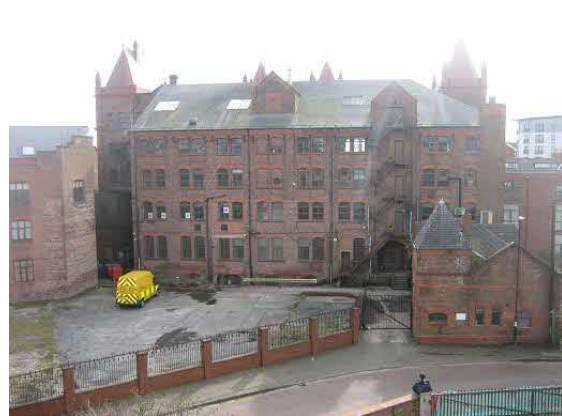
Figure 3: Rear (north) façade
