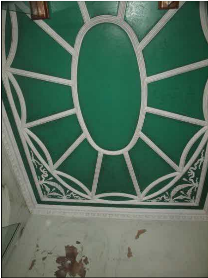
Plate 40: Ceiling detail, room 9
