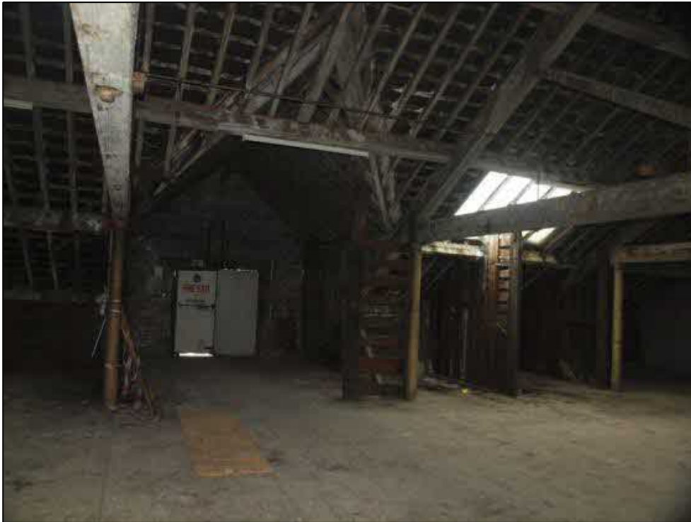
Plate 135: Room 6 showing fire escape
