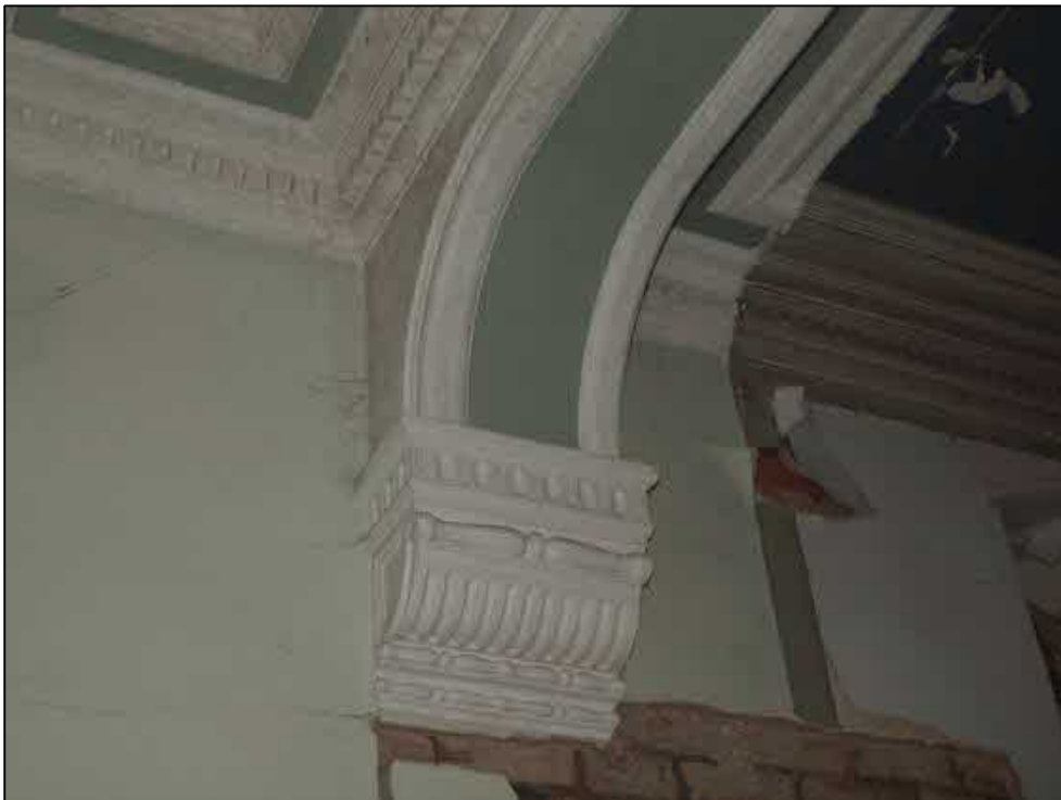
Plate 53: Detail of corbel
