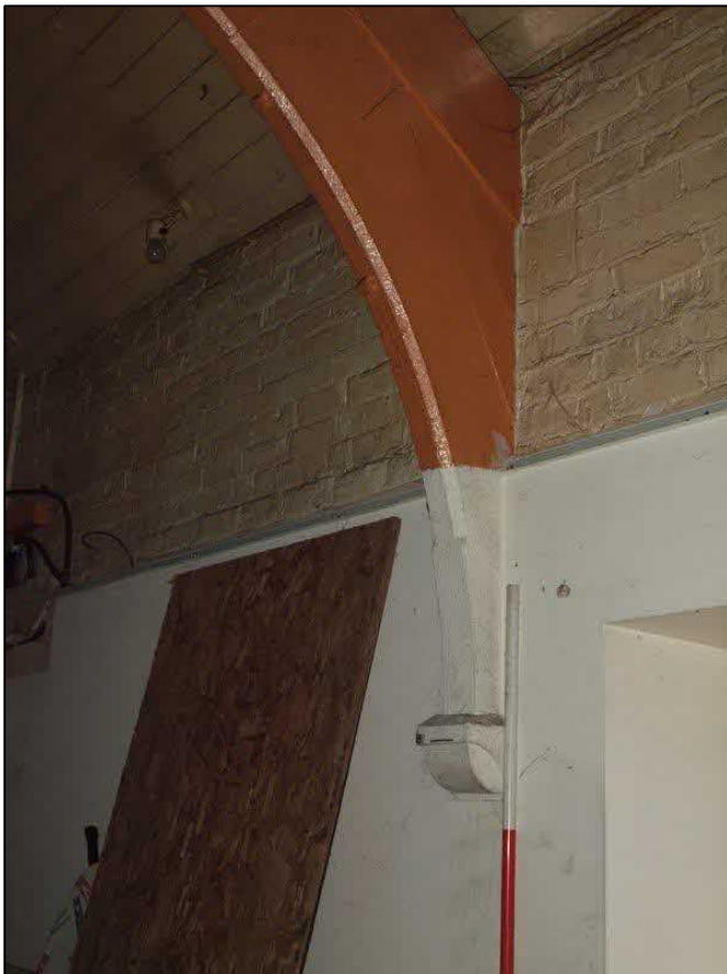
Plate 163: Detail of truss resting on corbel
