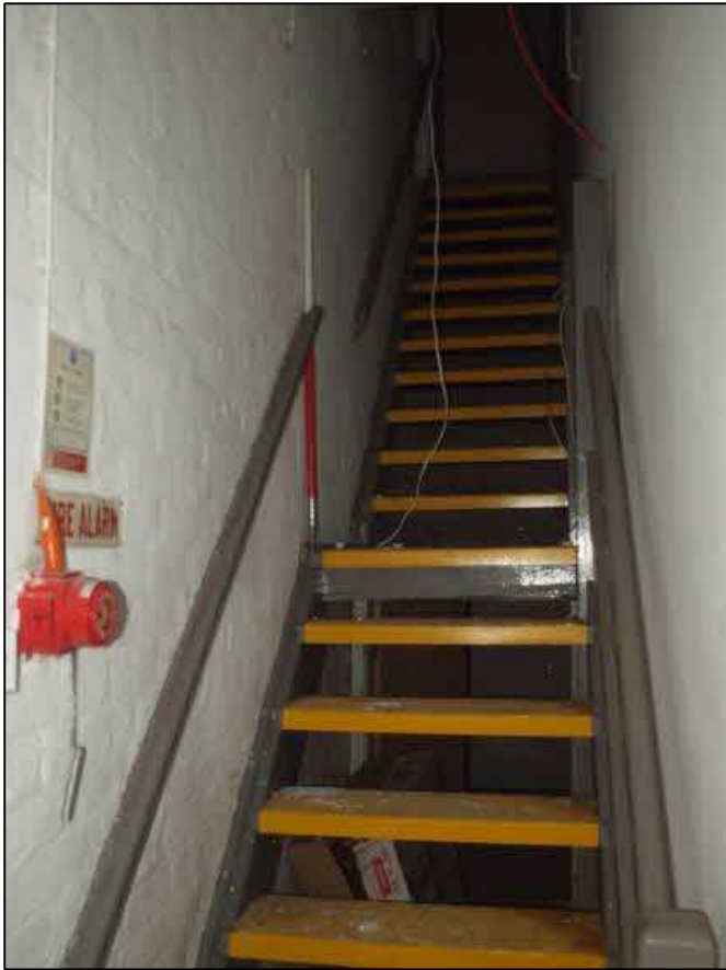
Plate 28: Inserted staircase between rooms 2 and 3
