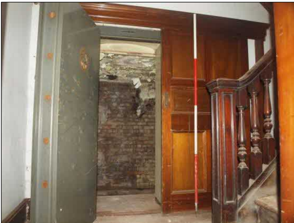
Plate 59: Doorway to room 18
