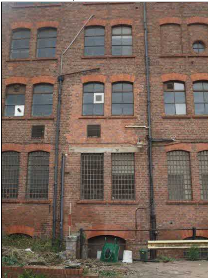
Plate 14: Bay 7 rebuilding at first floor
