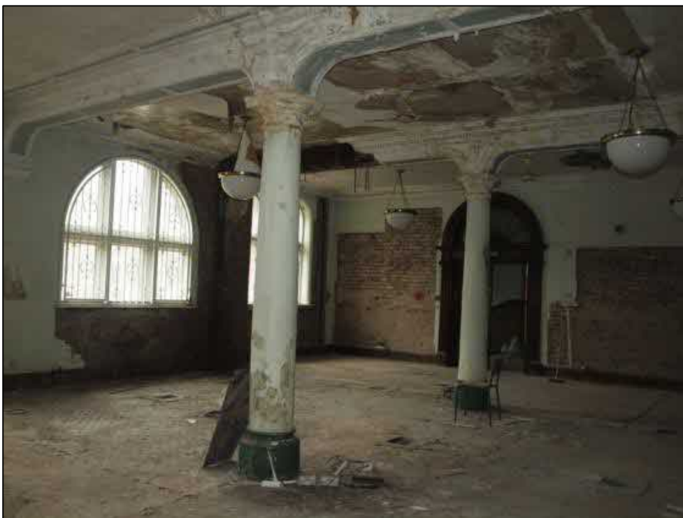
Plate 51: General shot of room 15
