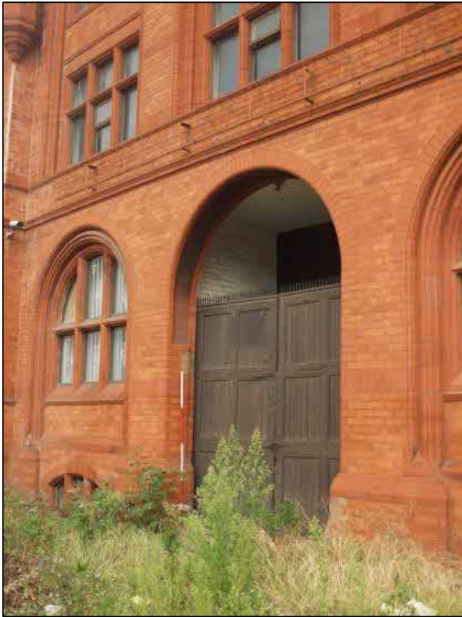
Plate 5: Detail of vehicle entrance in bay 3
