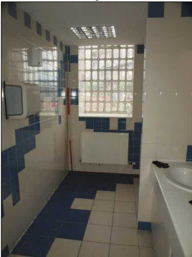
Plate 47: Inserted toilet block, room 13
