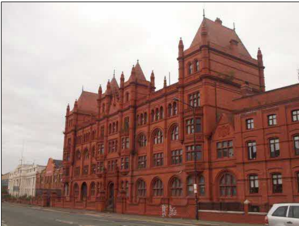
Plate 2: General shot of main frontage
