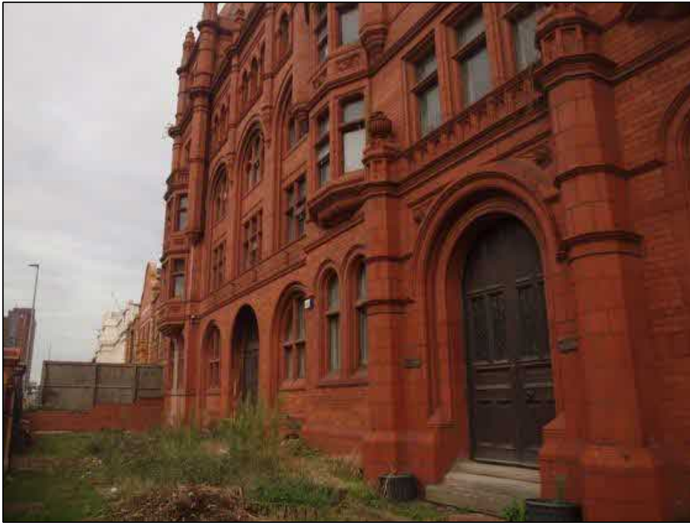
Plate 3: Detail of ground floor level
