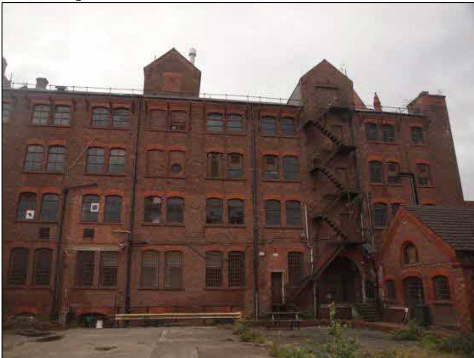
Plate 10: General shot of rear elevation
