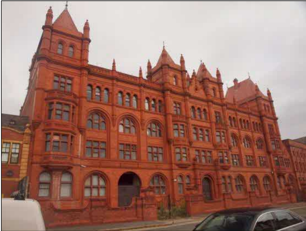
Plate 1: General shot of main frontage
