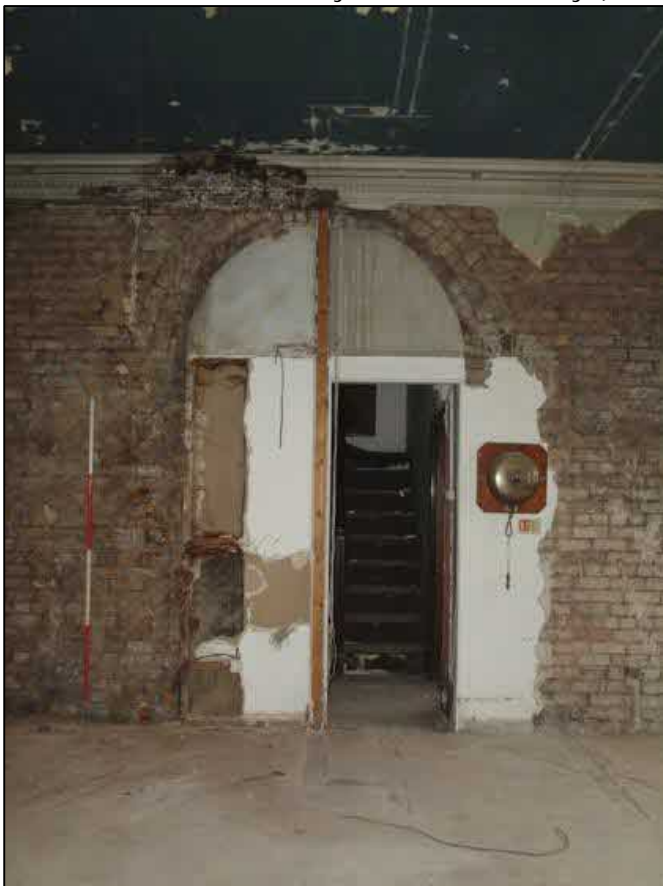
Plate 57: Detail of removed doorway and revealed opening to staircase (room 16)
