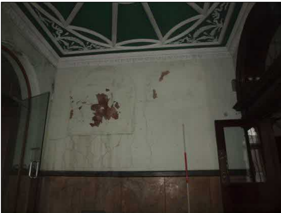
Plate 41: Blocked windows in room 9 onto stairwell
