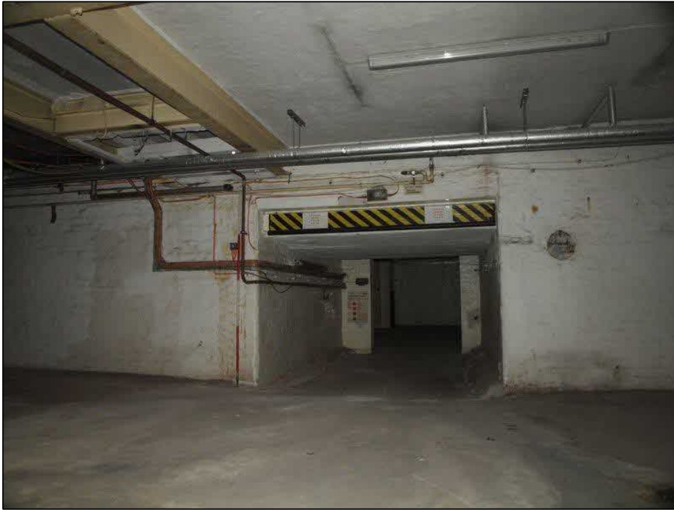
Plate 150: Room 10: Passageway below vehicle axes above
