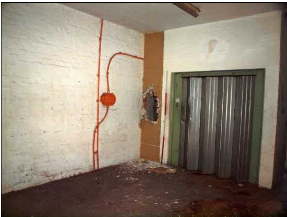
Plate 121: Room 5, inserted lift
