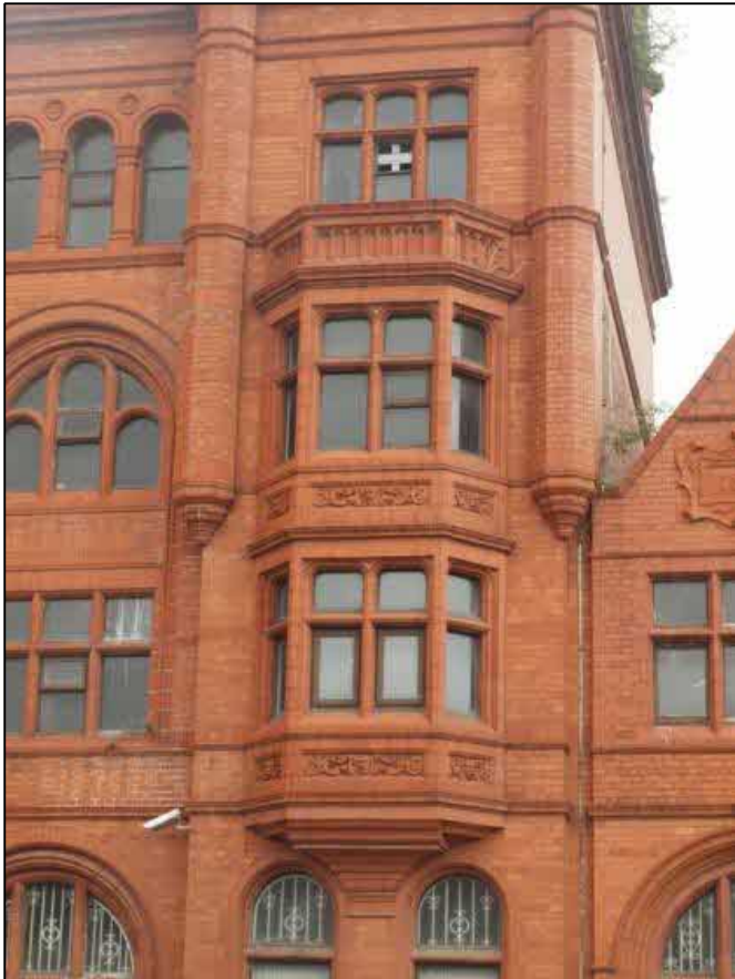
Plate 7: Detail of projecting bay window at first and second floors
