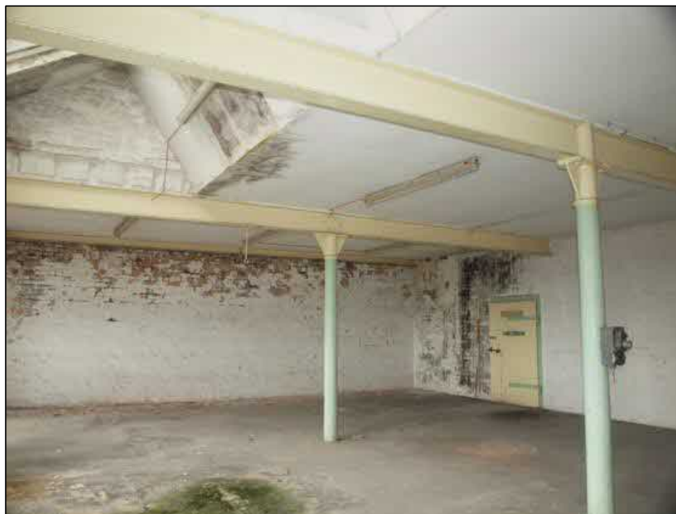
Plate 125: Room 7 showing change in ceiling and metal door
