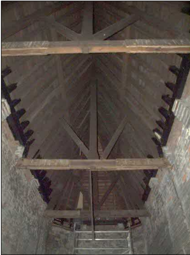
Plate 137: Detail of king post truss in room 7
