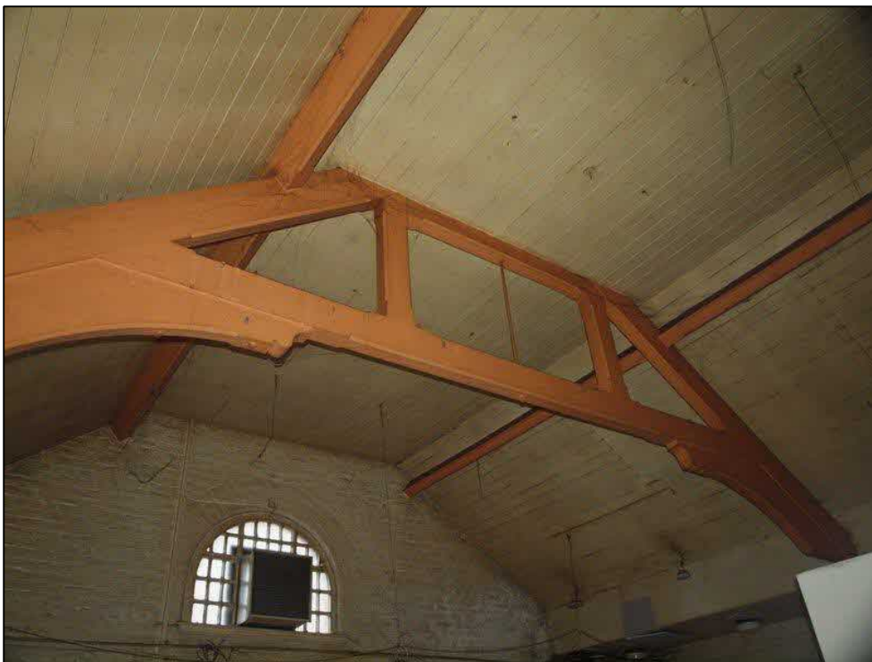
Plate 161: Detail of Queen post truss
