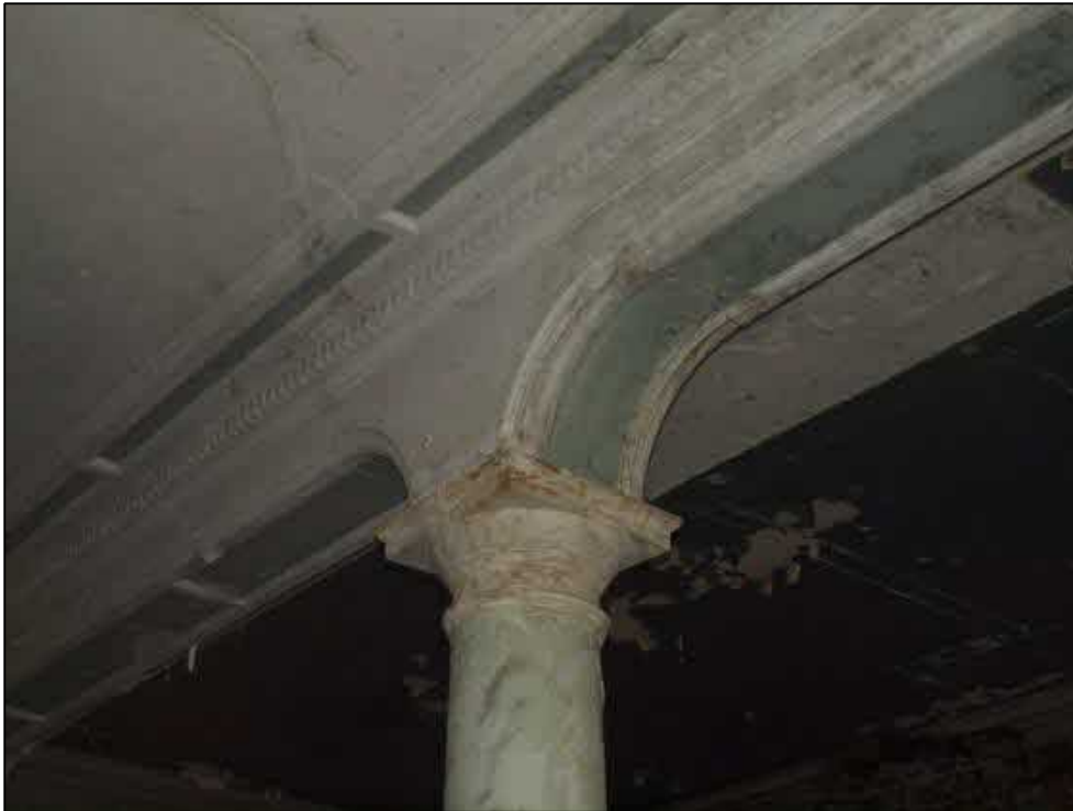
Plate 52: Room 15 detail of plaster on column and beam
