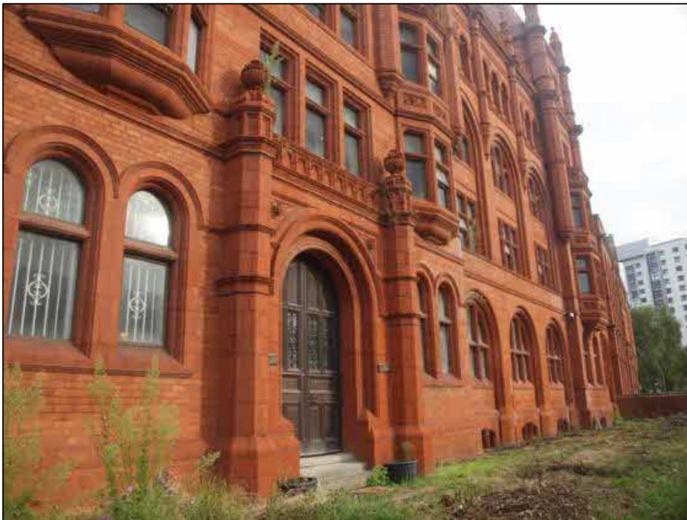
Plate 4: Detail of ground floor level
