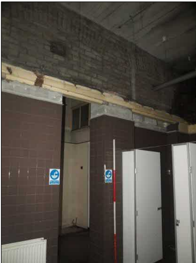
Plate 71: Room 23 showing blocked window high in the wall
