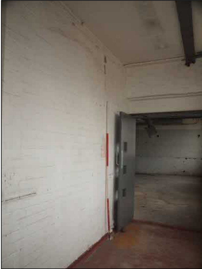
Plate 85: Room 8 showing blocked window
