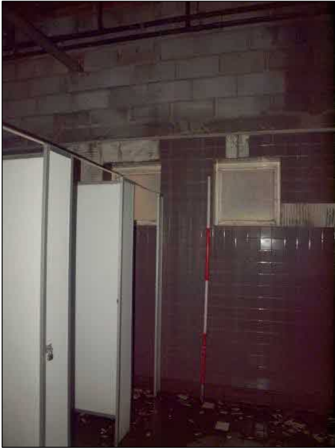
Plate 72: Room 23 showing concrete block construction
