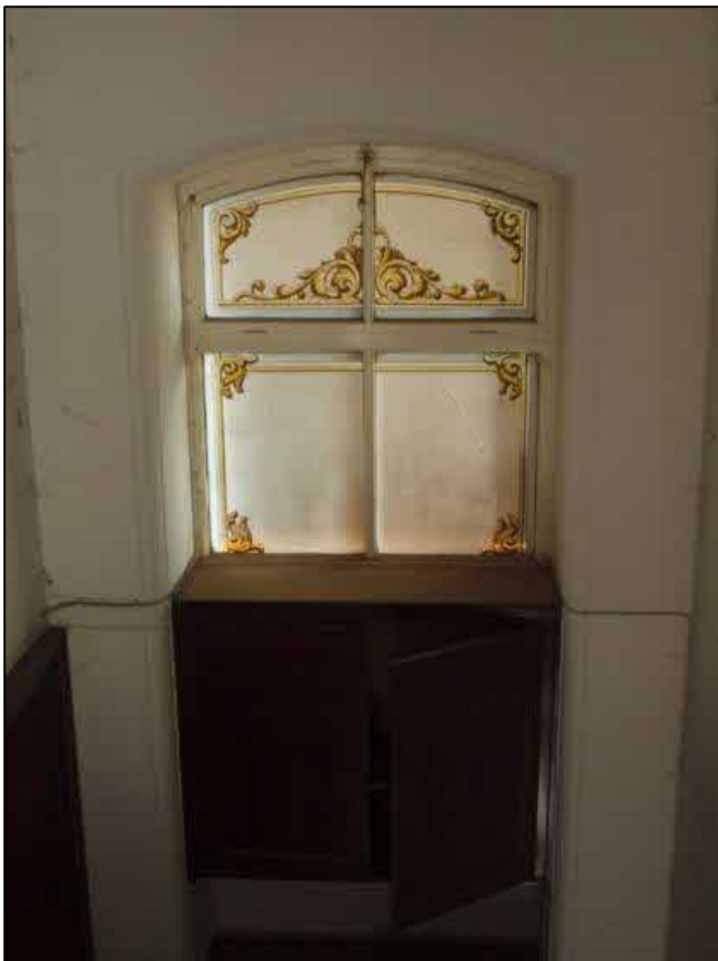
Plate 74: Frosted glass window on staircase
