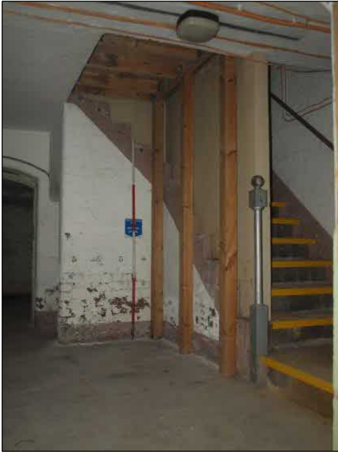
Plate 138: Room 1 main stairwell
