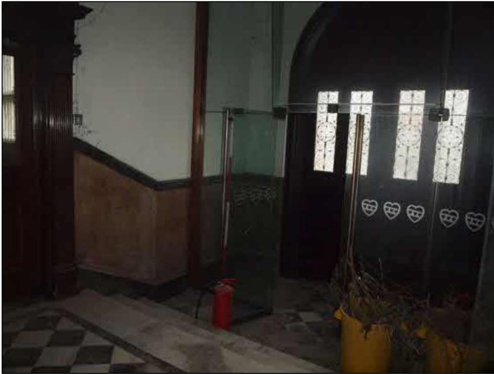
Plate 38: Main entrance, room 9 showing marble steps
