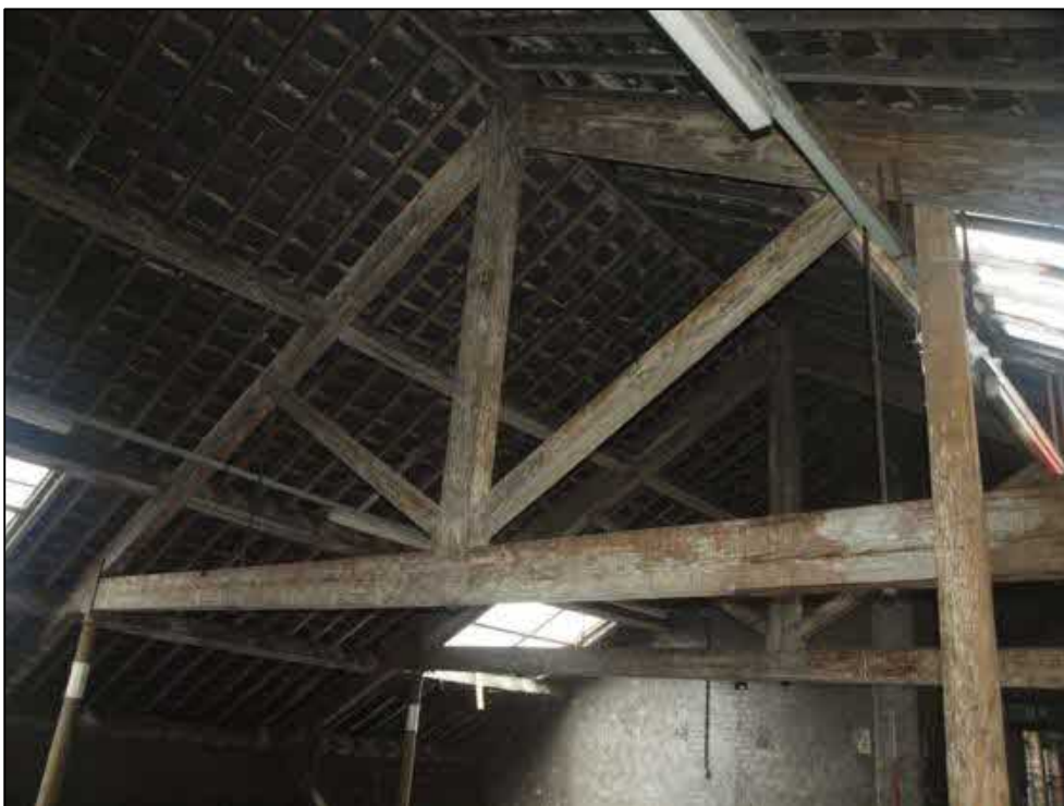
Plate 130: Detail of king post truss, room 3
