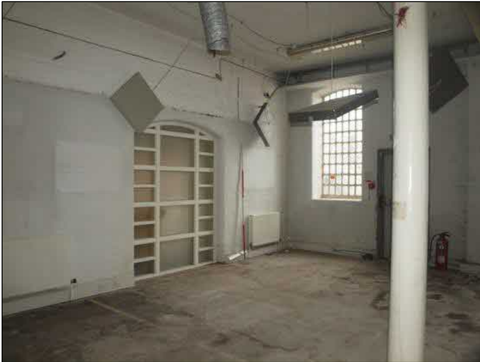
Plate 44: Room 11 showing window inserted into doorway
